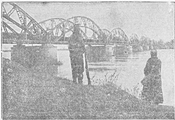
Ἡ σιδηροδρομικὴ γέφυρα τοῦ Ἀξιοῦ
